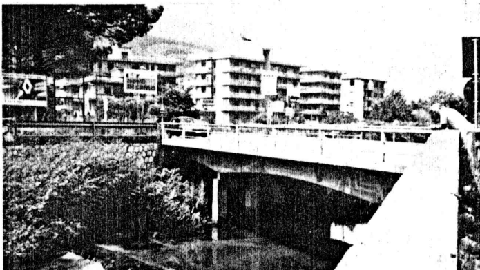
The bridge across the Rapido in the same area where Company "A" built their first bailey.
