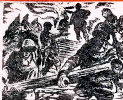
10 Back at the command post, Sorrell proposes blasting a tank road down the dry bed. No sale. At dark he is again put to building corduroy roads.
