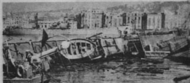
Naples harbor was heavily damaged.
