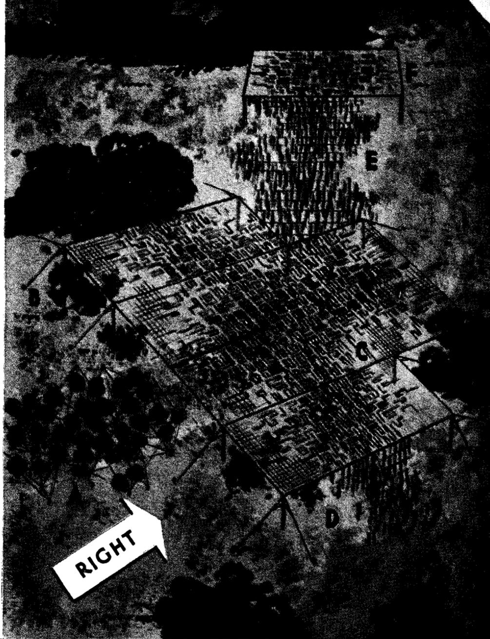
FIGURE 52 ②.—Dug-in position with supplementary camouflage. **A.** Irregular network of wire garnished with natural materials covers blast mark. Foliage changed after firing. **B.** Spoil darkened and textured with natural materials. **C.** Areas between nets garnished with 2-in. burlap strips. **D.** Net set tied in to existing foliage with garlands. **E.** Trampled areas concealed with garlands. **F.** Additional flat-top over supplies.
