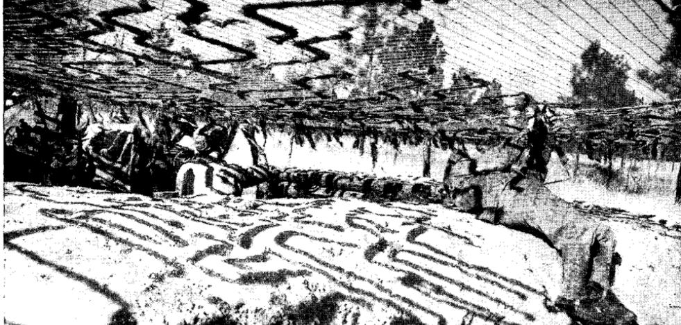
FIGURE 50.—Areas between nets *must* be garnished with additional burlap strips or textured patches.
