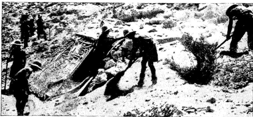
FIGURE 14.—British 25-pounder position located against an escarpment. Use was made of dummy stones in blending position with background.
