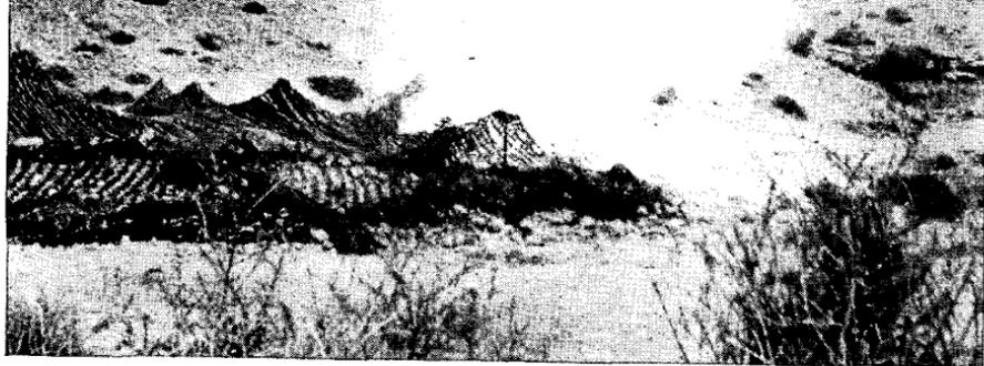
FIGURE 13.—Gun in action. Except for embraiture, camouflage remains in place. Embraitures can be closed quickly after fire mission is complete, or, if piece is moved, drape can be removed quickly.
