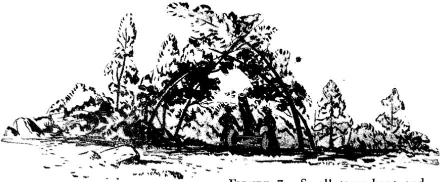
FIGURE 7.—Small trees bent and wired together over gun position.
