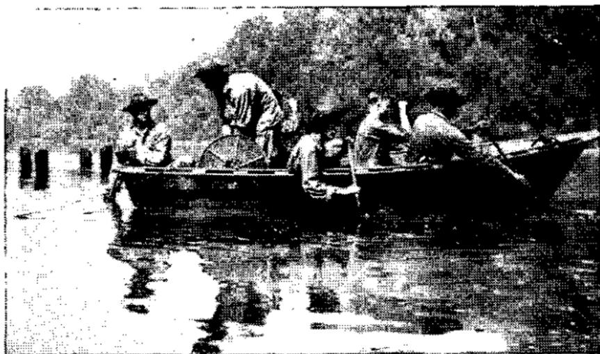
FIGURE 45.—Assault boat used to carry anchor cable across stream.
