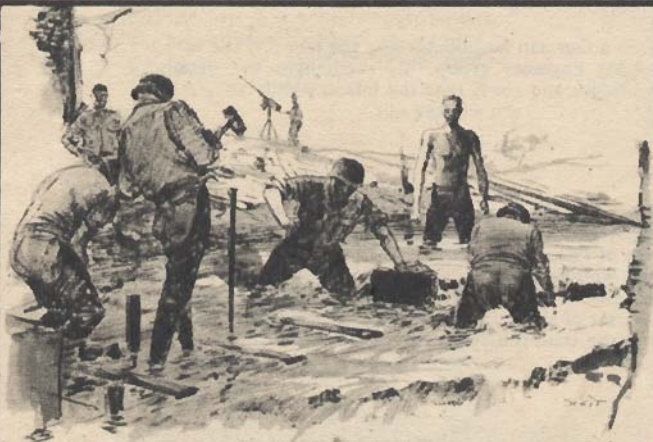
Engineers, above, working in a swiftly flowing stream preparing the seating for a bridge trestle. This is near Gulpin in Holland. Below, the trestle bent being lowered into place after the bed of the stream has been made ready for it.
