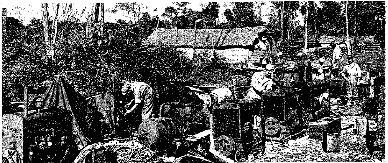
Air Compressors Salvaged from the Beach at Rangoon, being Reconditioned at an Engineer Depot in Assam
