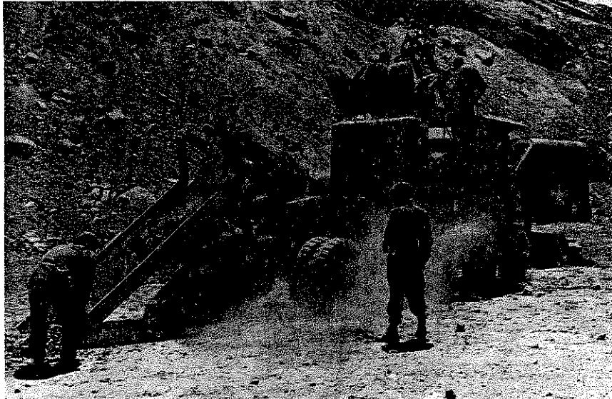
Engineer Troops Using Rock Crusher in Road Construction Work in North Africa
