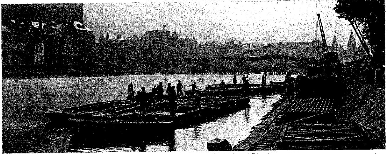
Construction Work on the Floating Bailey Bridge at Dinant
