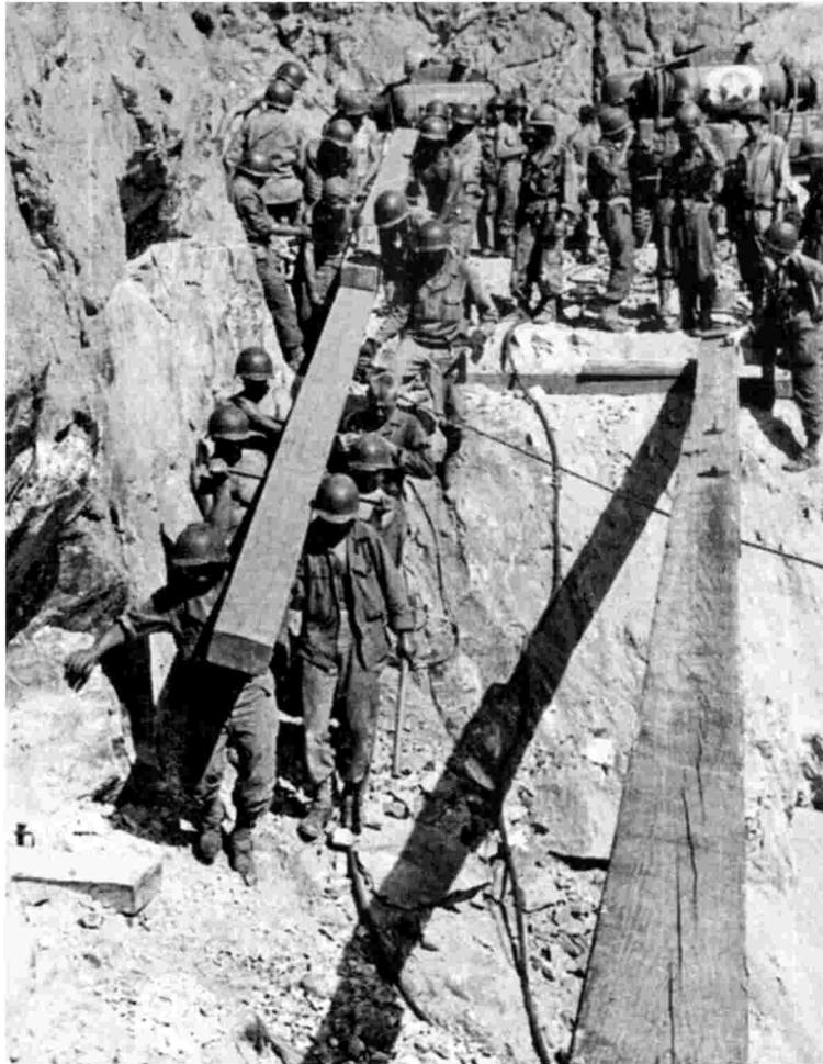
over. But it held, and nothing else mattered. When the vital spearhead of the division got across, traffic was halted again and the engineers were given three hours to strengthen the bridge for heavier traffic. A third heavy upright inserted in the middle of the span would do the trick.
