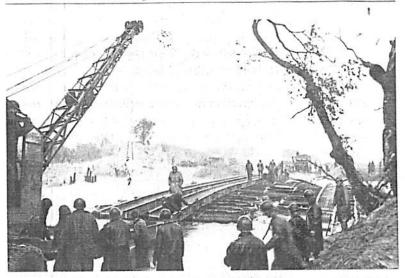
The 16th Engineer Battalion adds steel sections to protect a ponton bridge against the rising waters of the northern Volturno River.
