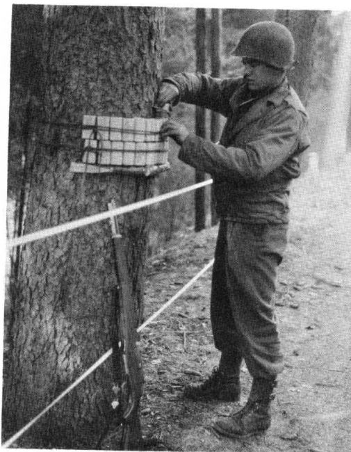
PLACING CHARGES TO DROP TREES across roadways.
