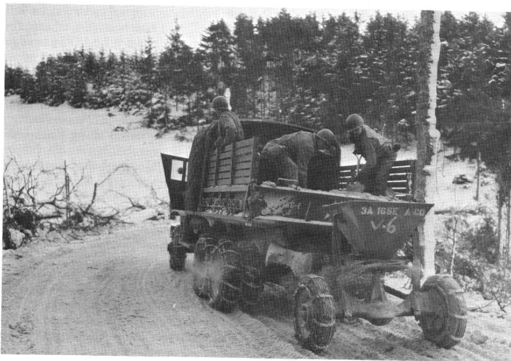
ROAD MAINTENANCE OUTSIDE WILTZ, BELGIUM
