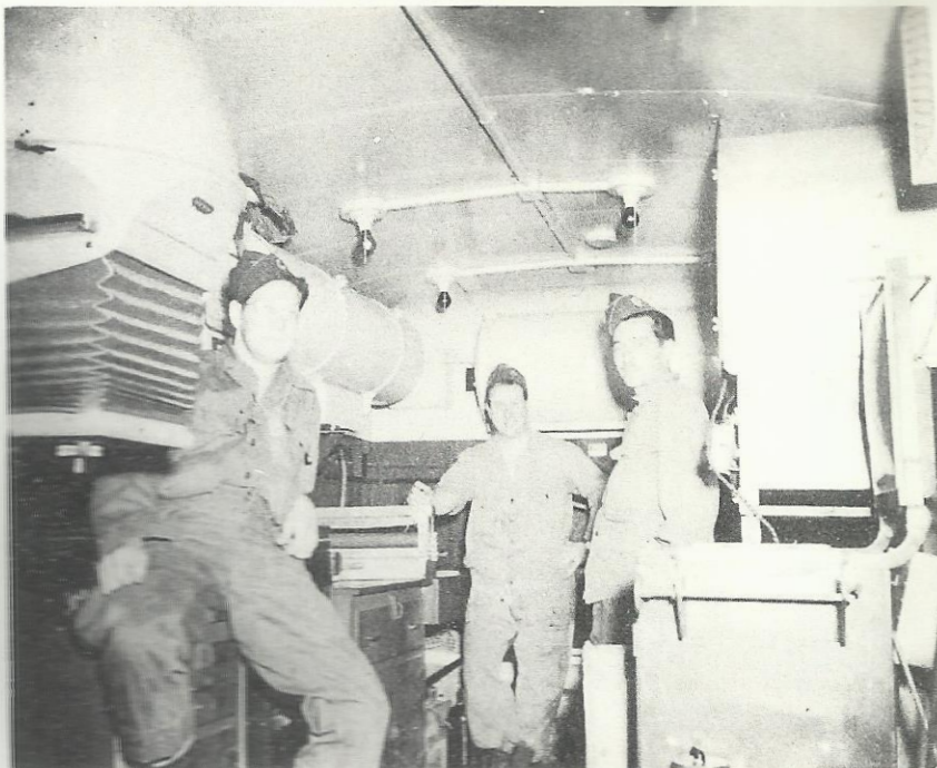
This van, containing a photo-finishing section complete, was acquired by the company in February '45. These men work with contact printing frames, photo-enlarger, developing tanks, and print drying machine.
