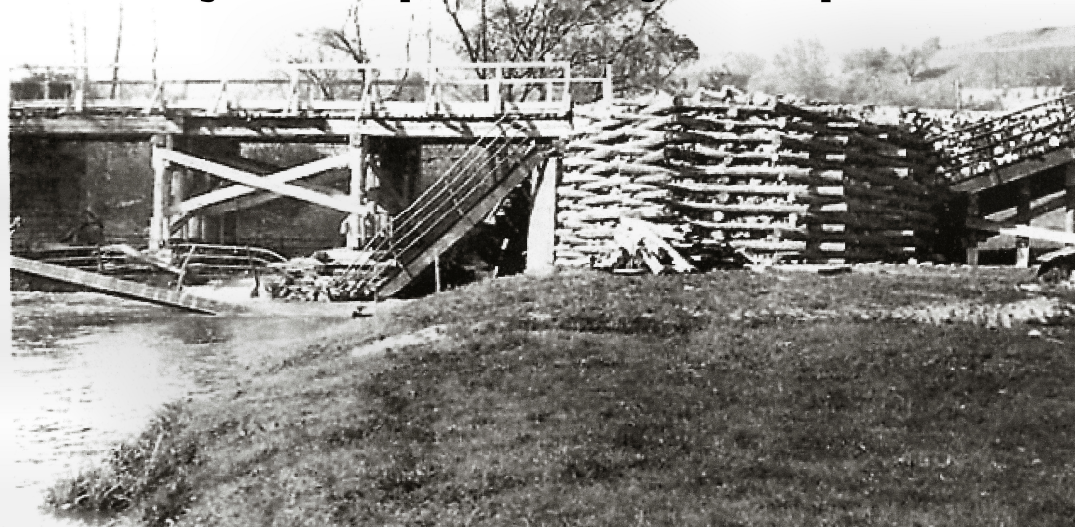
----- Last Bridge built by Co B 48 Engrs., 4 May 1945
