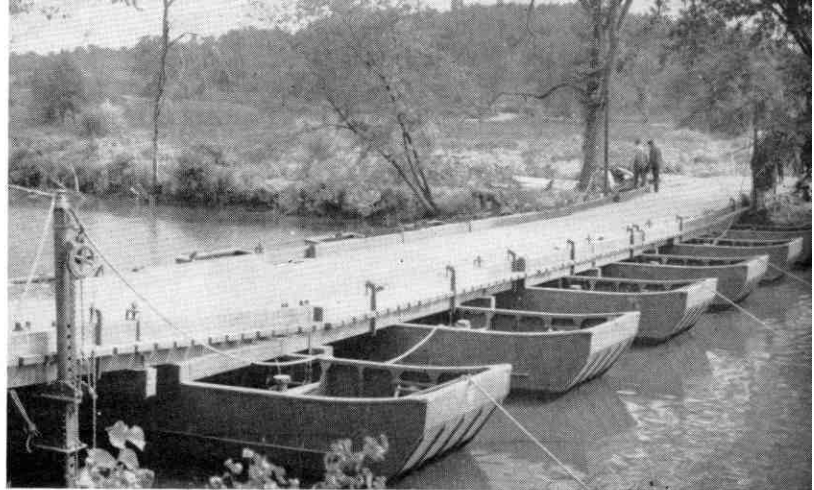
Bridge over Stillwater River, Fort Devens.
