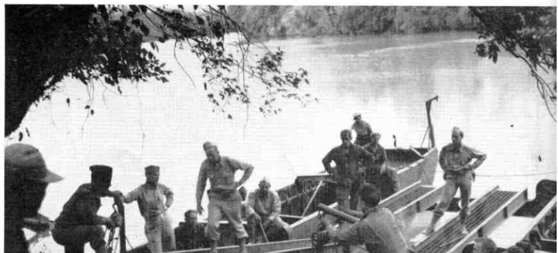
Approach runways in position.
