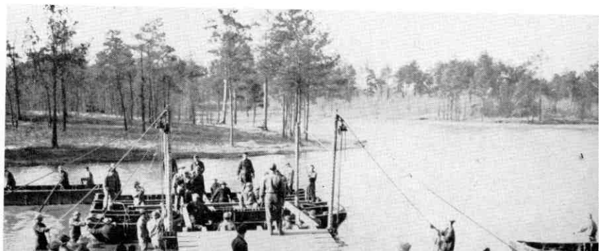
General view of bridge over Mac Faydens Pond.
