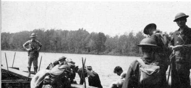
Foot bridge at Macomb Reservation.
