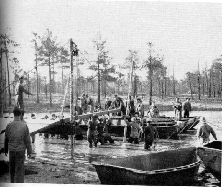
Men place trestles in position.
