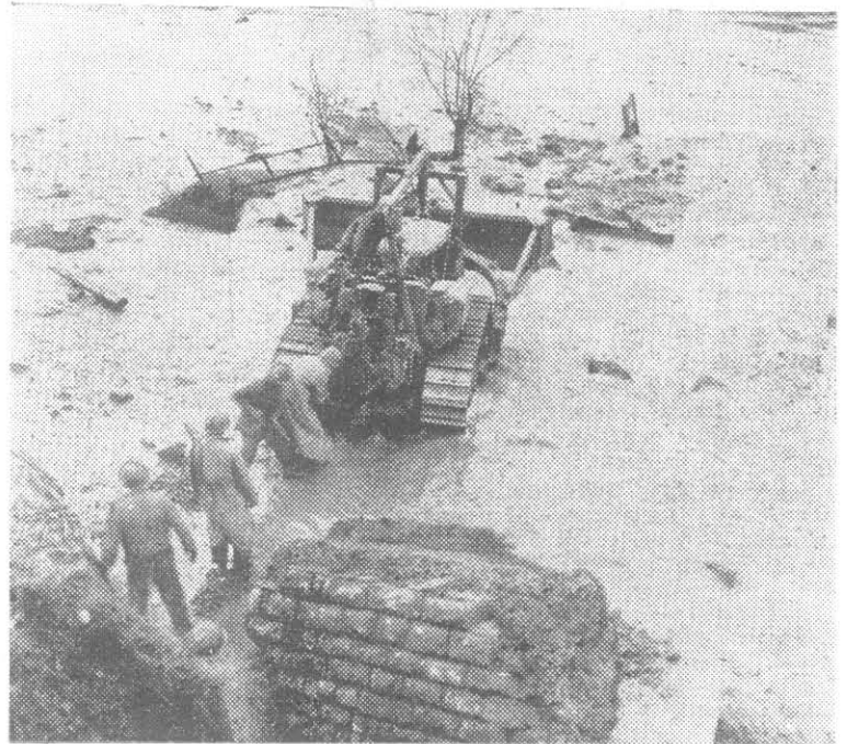
Maybe they'll cuss it sometimes, but the engineers are quick to expound on the merits of the bulldozer. This one, used by the 36th, sits in water while GIs attach a chain around a large concrete block to be pulled away. The flood was caused when the hurrying heinies blew some dikes.
