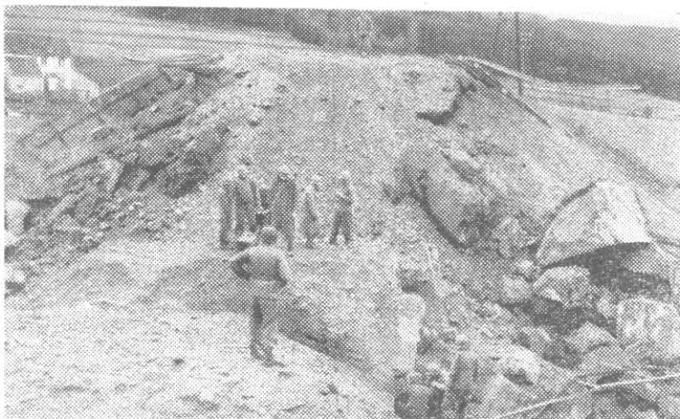
It's another kraut-blasted bridge, dynamited in such a way to cause a headache in road block form. But it's a headache the 36th GIs are going to remove, using TNT in lieu of aspirin tablets.
