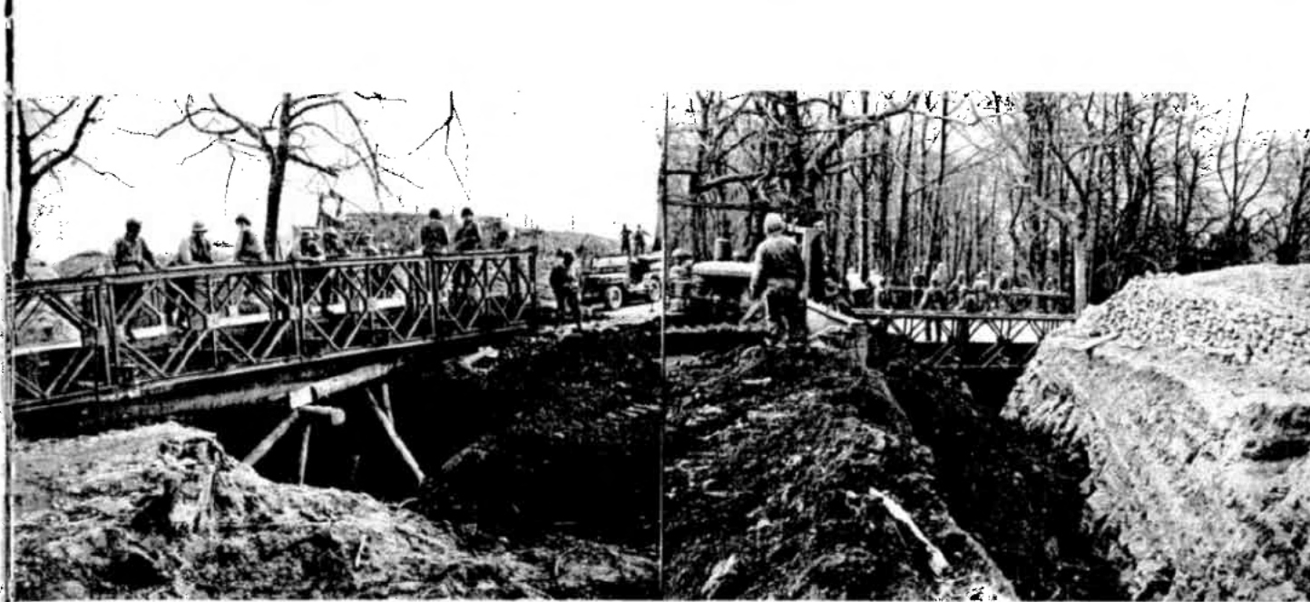
DOUBLE-SINGLE BAILEY OVER ANTI-TANK DITCH
