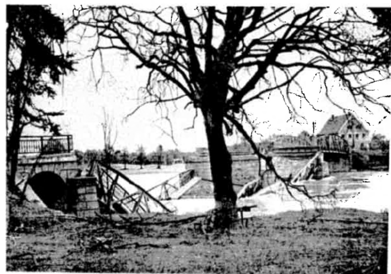
Blown Lovingen Bridge over Danube
