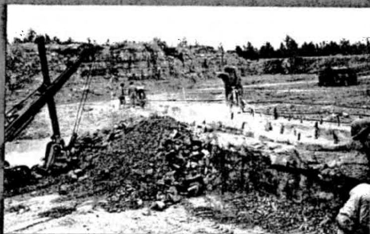
ONE OF THE MAIN JOBS WAS QUARRY OPERATION
