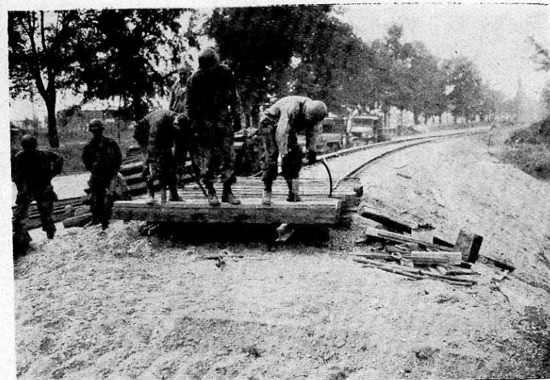
Laying track at the approach to Charlie Company's bridge, Mannheim, Germany, August, 1945.
