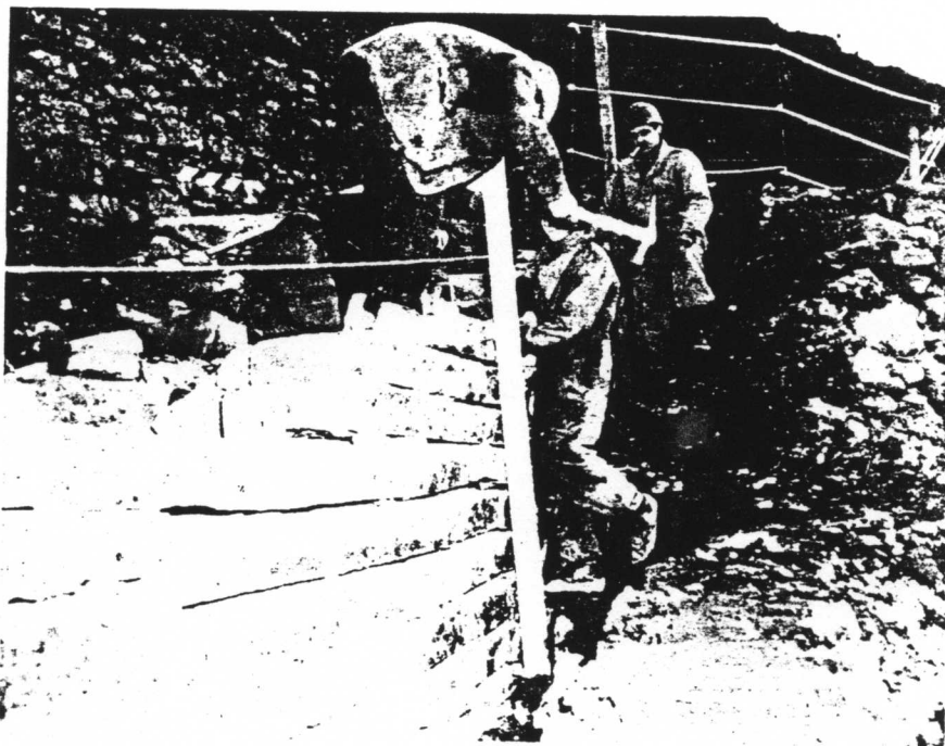
235TH CORPORAL SUPERVISING WORK OF ITALIANS NEAR POPIGLIO
